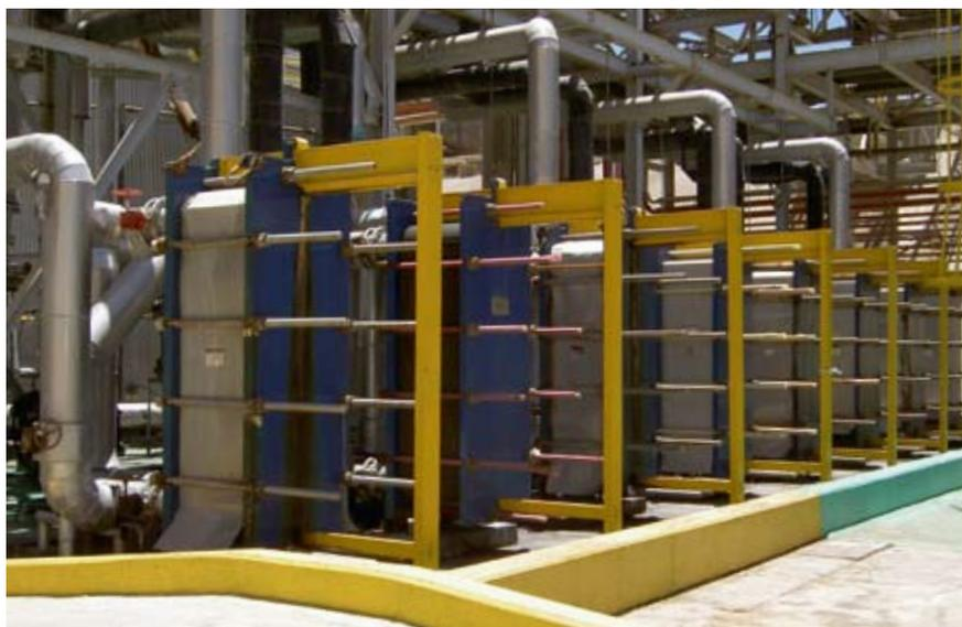
Six of the 16 heat exchangers at the Barrick Zaldivar copper mines in Chile. The mechanical construction of the Alfa Laval Plate heat exchangers makes them easy to open and clean by unscrewing the tightening bolts.
